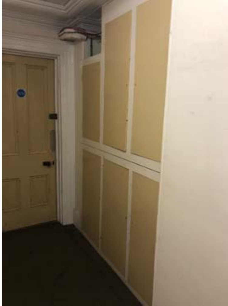
(view from southwest)
