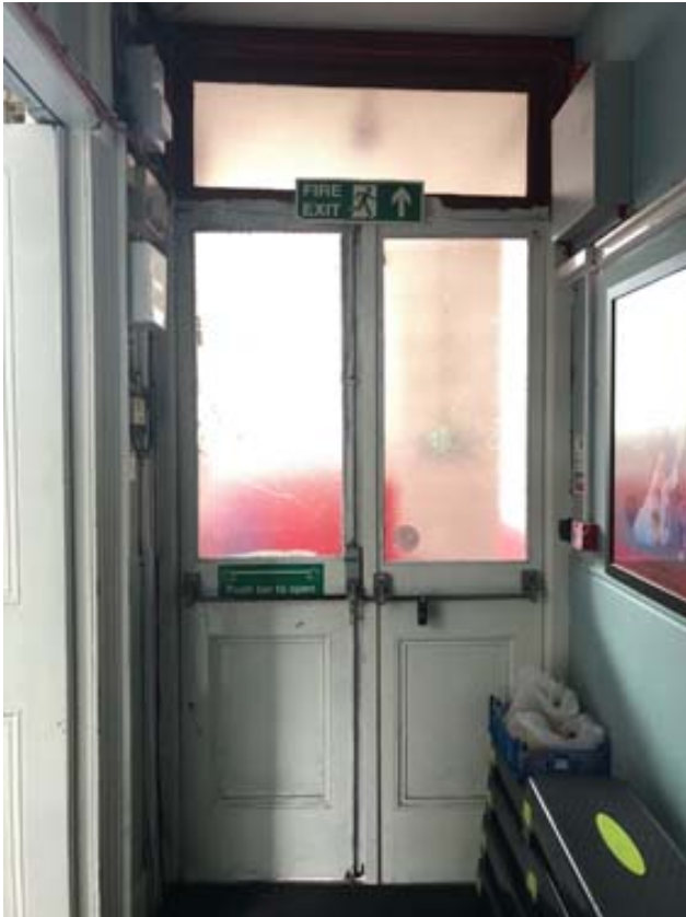
(view from west)
